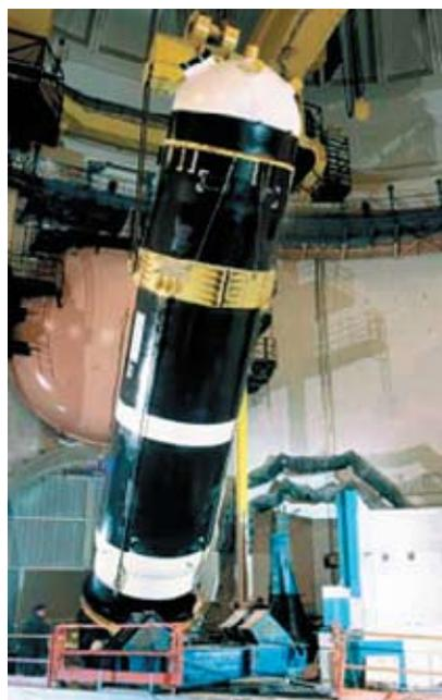
Figure 3.17 - Erection of a Pressuriser in a reactor building.
